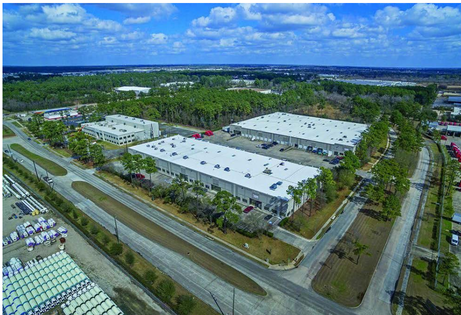
Jud Haggard/Courtesy of HFF Interwood Business Center
